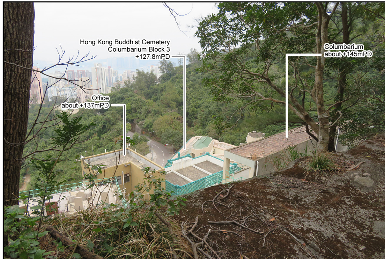
VIEW FOR EXISTING CONDITION
