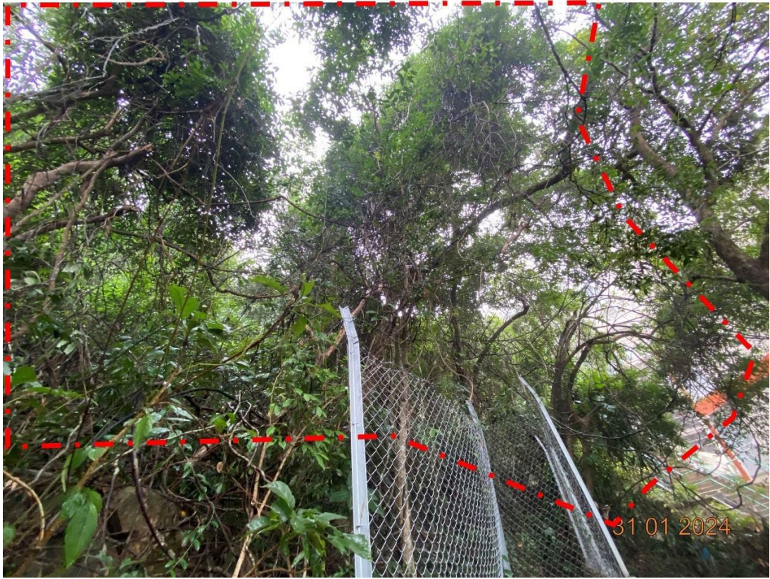
V27 : General view of TG2
